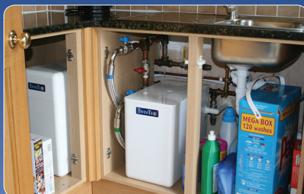
The TwinTec installed under a kitchen sink.
